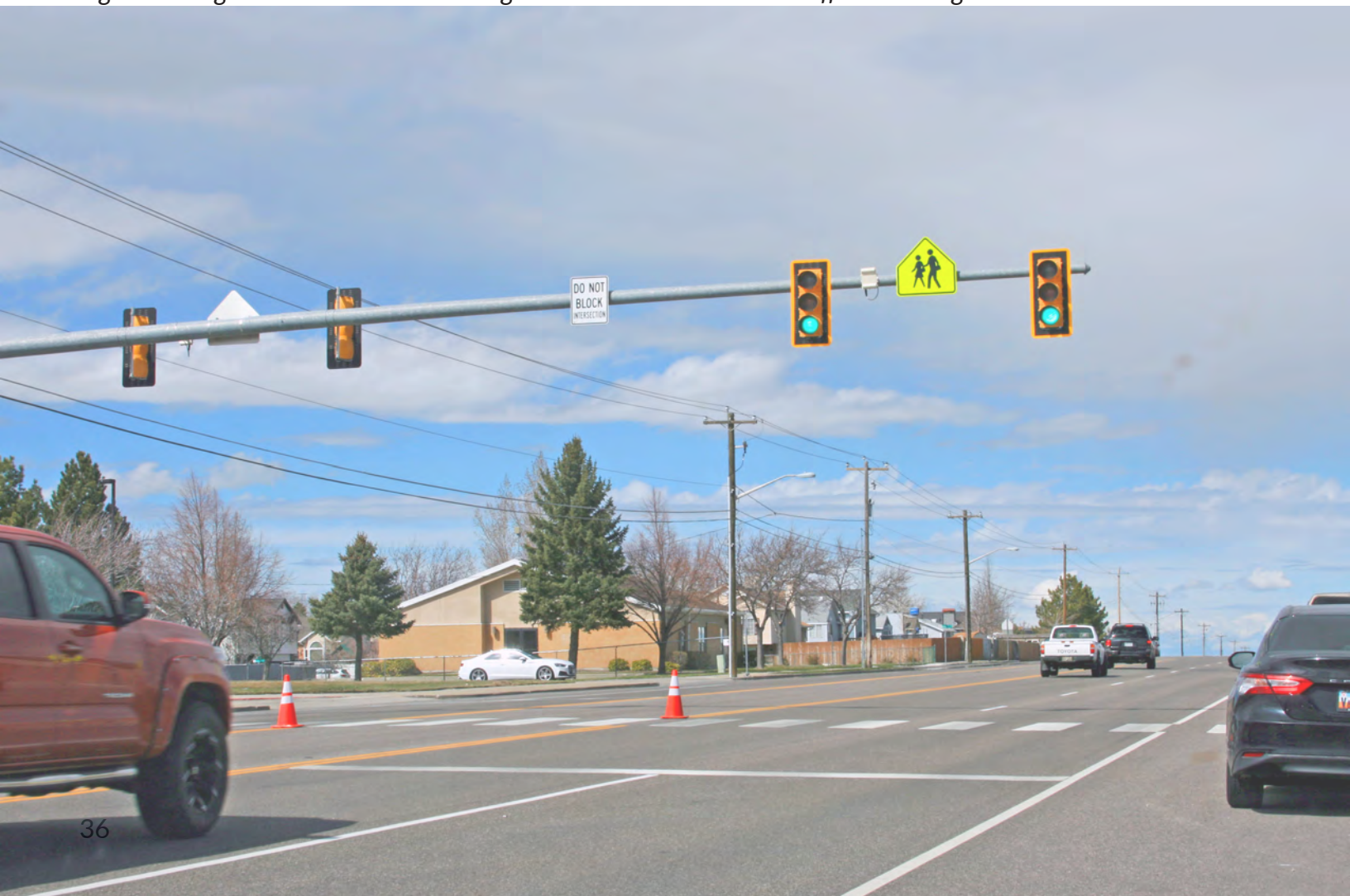
Figure 6.1 Signalized mid-block crossing on 5600 W near Thomas Jefferson Jr High School.
