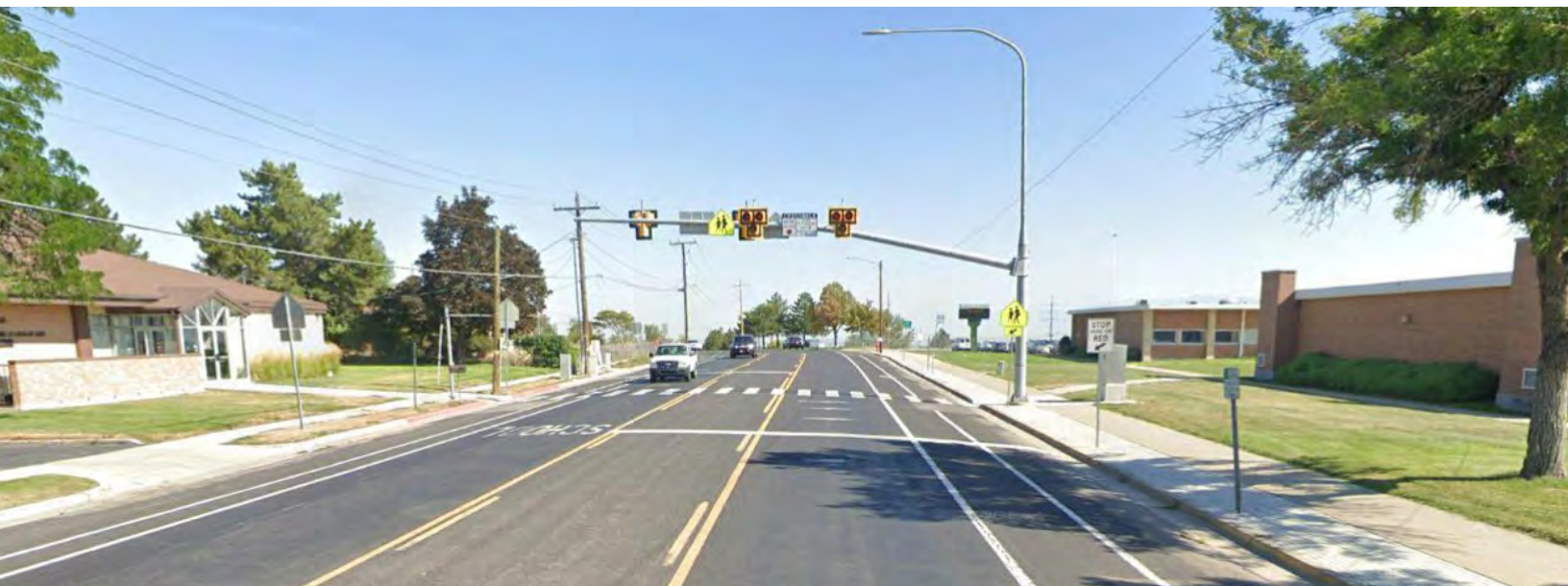
Figure 1.1 HAWK crossing on 5500 S Cougar Ln. in Kearns.
